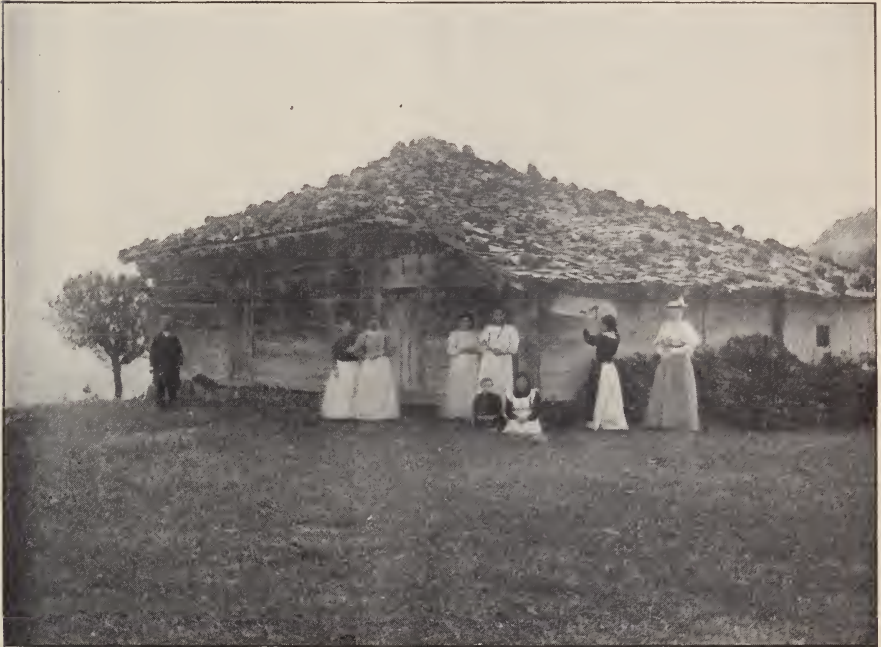
THE OLD KAPOU KAYA CHURCH Roof covered with stones
